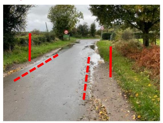
**Detail:** Install cobbled strips along this stretch, hatching them in, to slow drivers down before entering 30mph zone and main built-up areas of Rodington. Location: **///informed.disbanded.stays**
